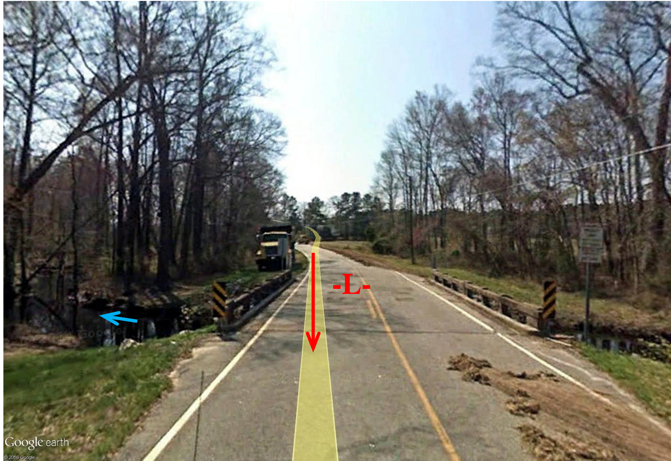
Looking South towards End Bent 1
